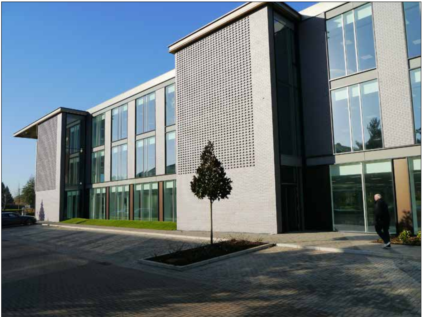
Croxley Green Business Park, near Watford, was designed by ESA Architecture
